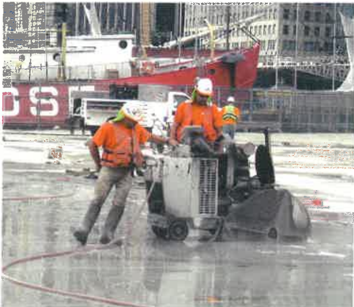
The pier deck was cut into sections using flat saws, some cuts being as deep as 18 inches.
