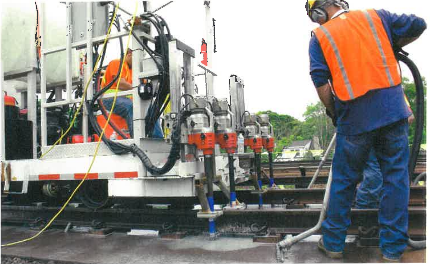
Slurry created during the drilling work was controlled by wet vacuums.
