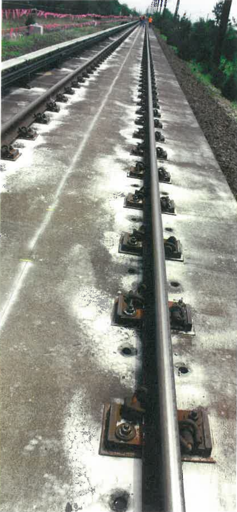
All 23,680 core holes were completed in just nine weeks.
