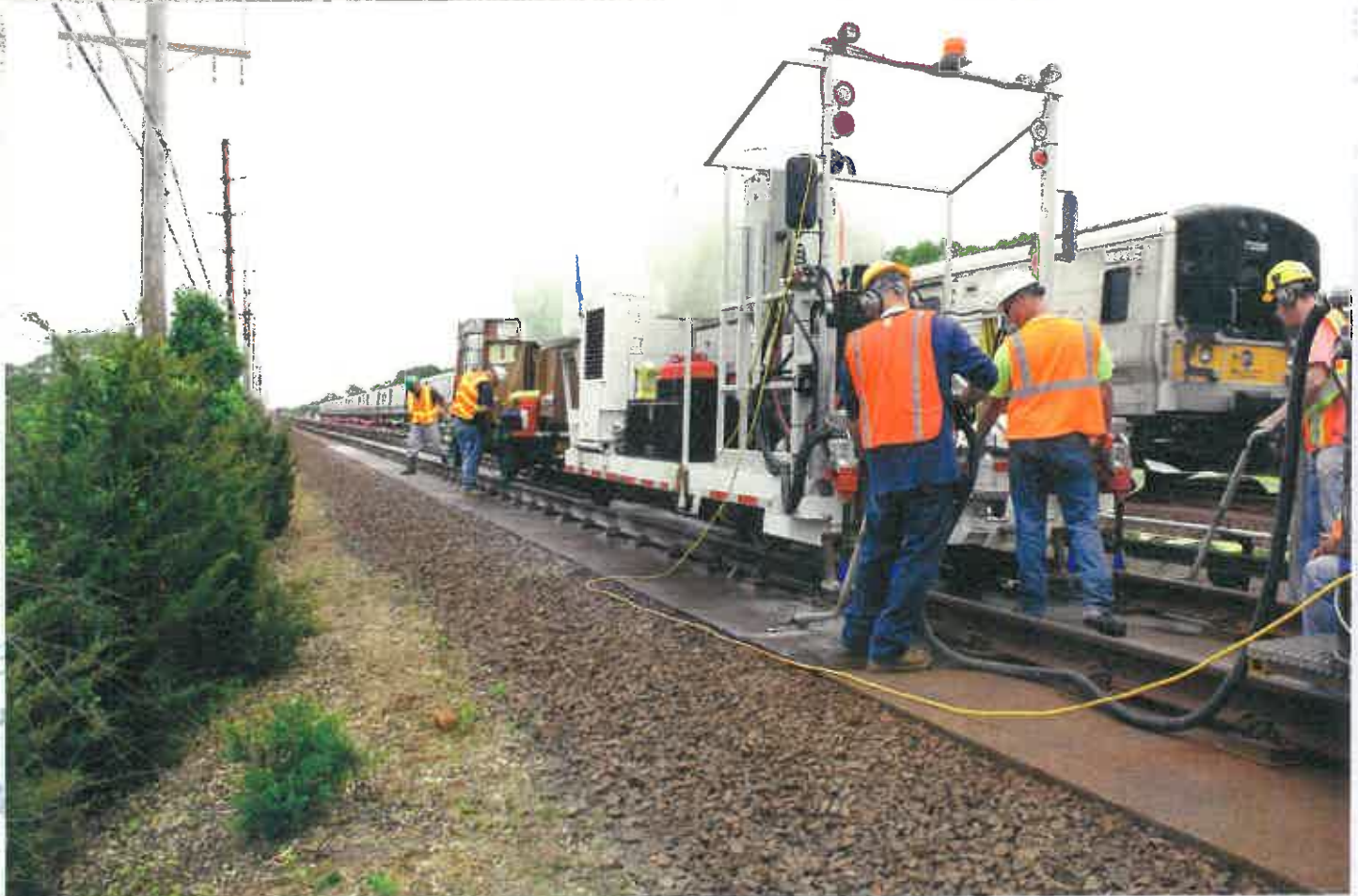
The contractor created a custom drilling machine dubbed the LIRR Railcar
