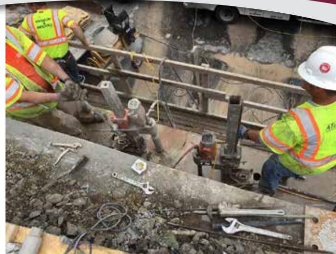
Atlantic workers core drill new anchor bolt holes in the existing bridge abutment.
