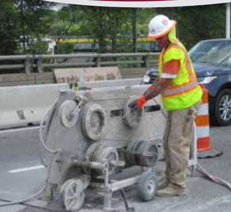
Scott Conaway prepares the wire saw for cutting through bridge diaphragms.
